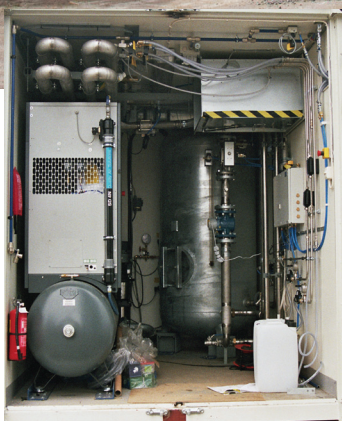
Serviceroom: compressor, flow meters, watertank and additive tanks
